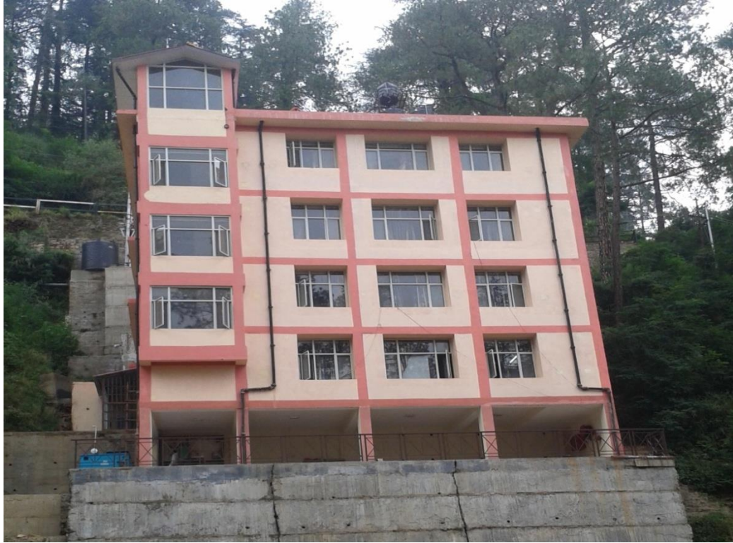
Divisional Data Center, Shimla
