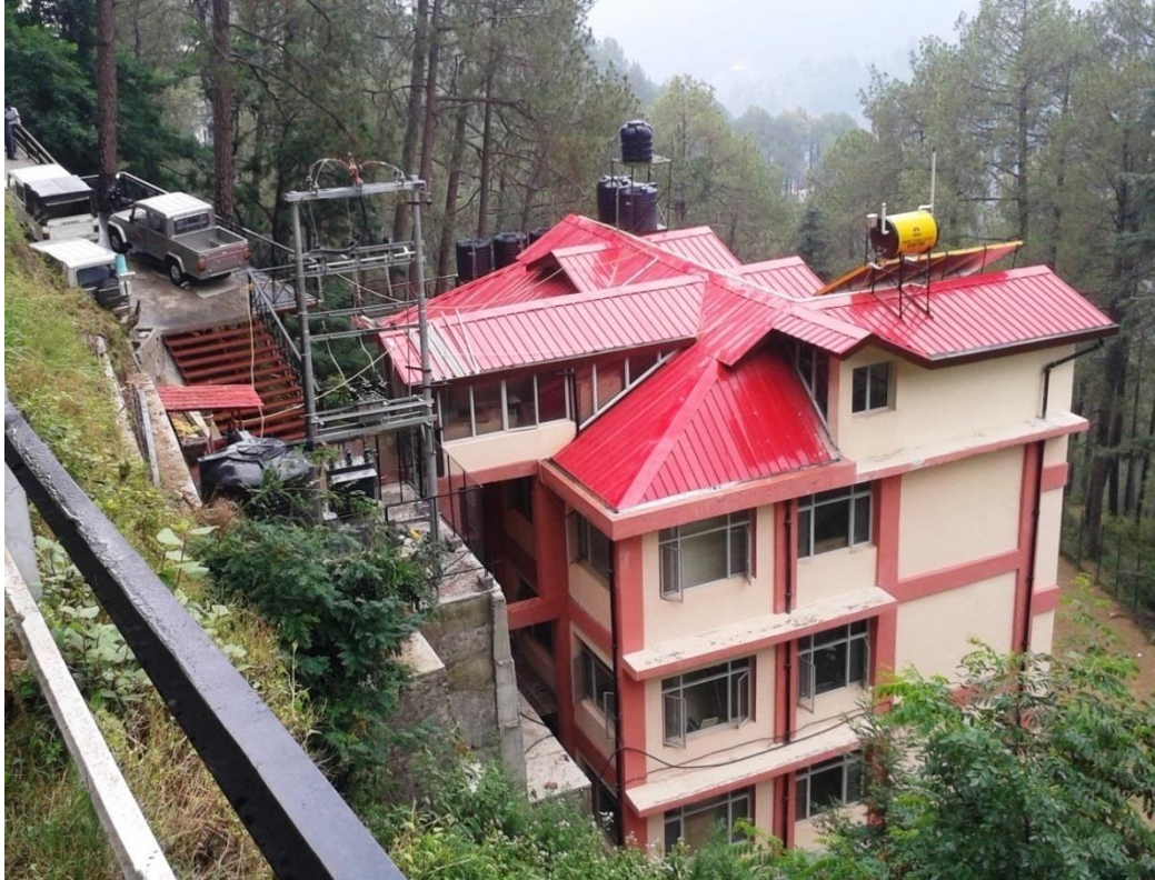
Divisional Data Center, Shimla
