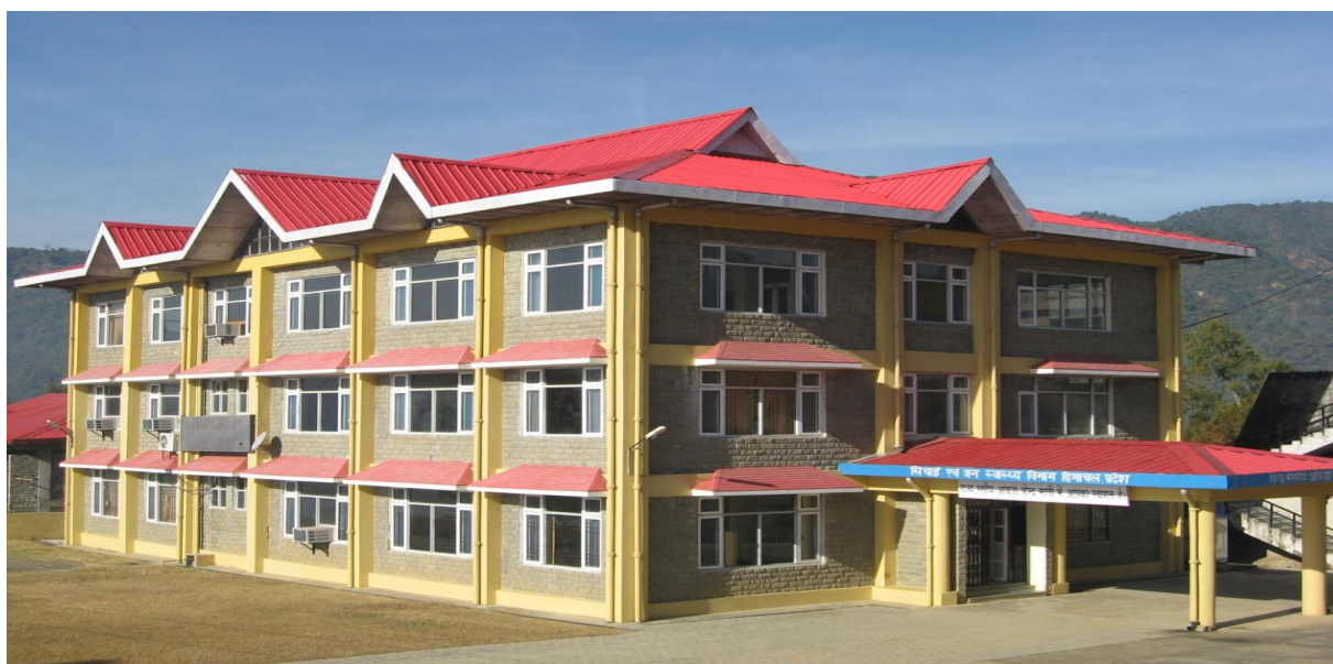
State Data Center, Mandi
